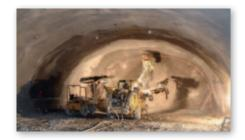
Machine Positioning and Control Drilling carriage, DIBIT™ tunnel scanner
