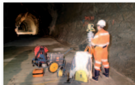
Geodetic Control Measurements
